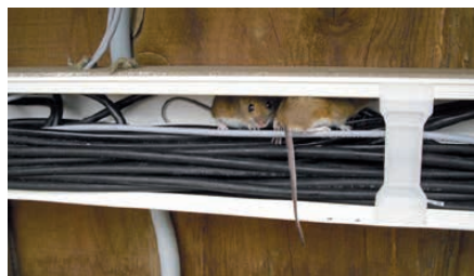
Cable ducts are designed to protect cables from damage; improper installation will cause problems.
